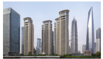
Tomson Riviera Apartment Towers Shanghai, China
