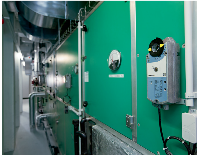
Powerful OpenAir damper actuators for HVAC applications – from 2 to 35 Nm and from 125 to 250 N.
