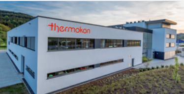
Headquarters (5.300 m 2 ) in Mittenaar-Offenbach (Administration and Production)
