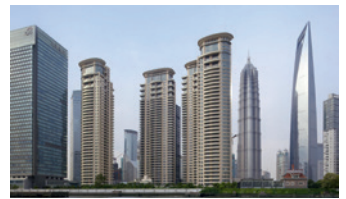
Tomson Riviera Apartment Towers Shanghai, China
